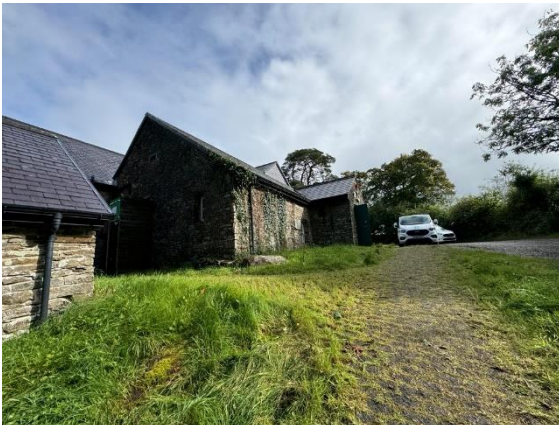
Figure F.15: u1b5 Buildings
