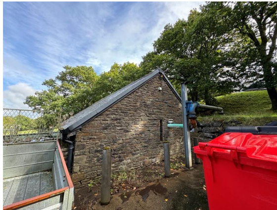
Figure F.16: u1b5 Buildings
