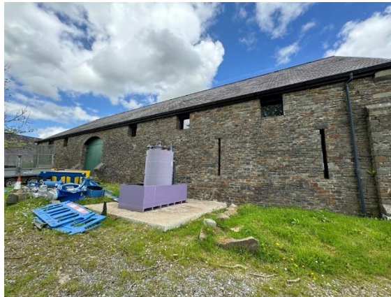
Figure F.14: u1b5 Buildings
